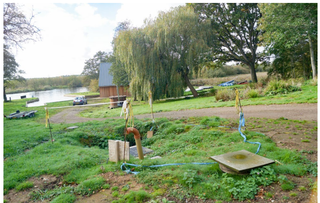
The height up to the water treatment plant is 65m and 4m in height. This plant couldn't be installed closer to the river due to the instability of the wet grounds.
